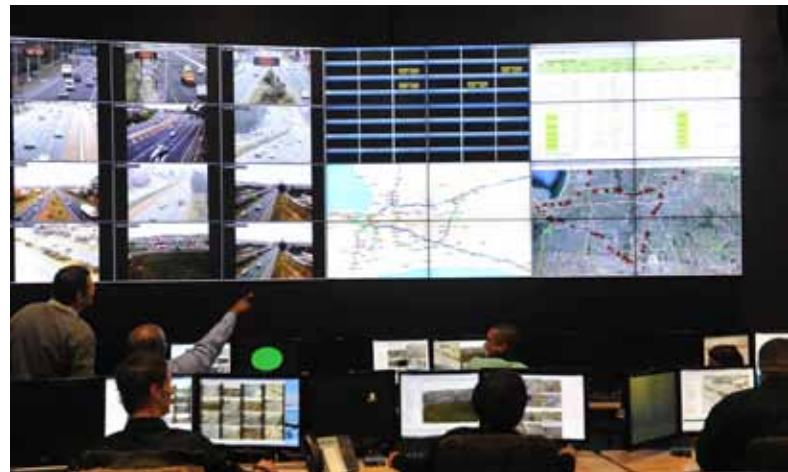
The City's integrated transport centre, a first in South Africa
