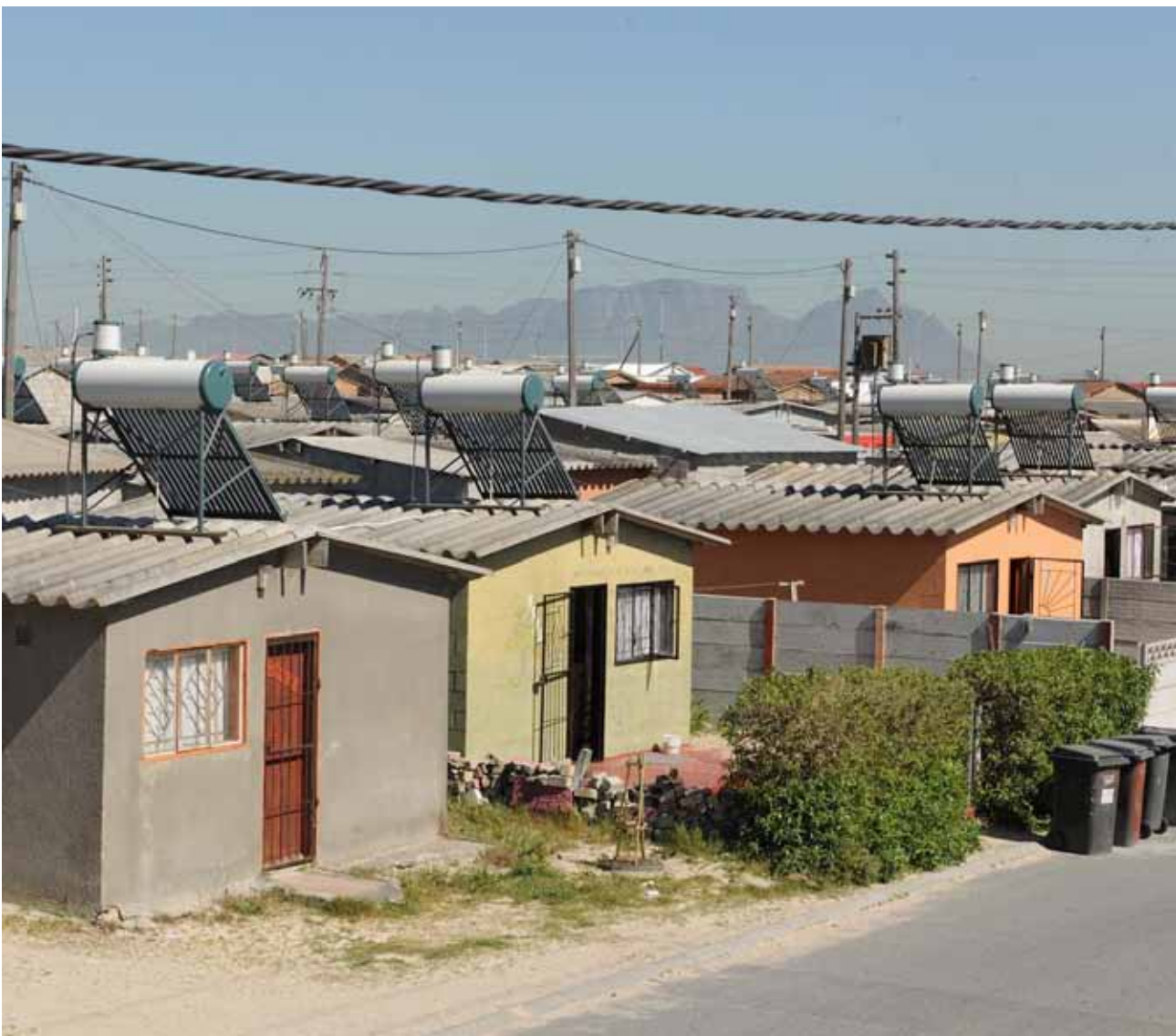
The pioneering Kuyasa housing project provided over 2 000 households with energy-efficient solar water heaters, lighting and ceilings
