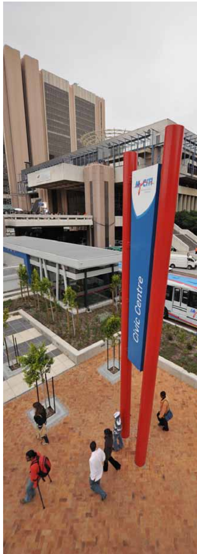
Cape Town Civic Centre and the new MyCiti bus station
