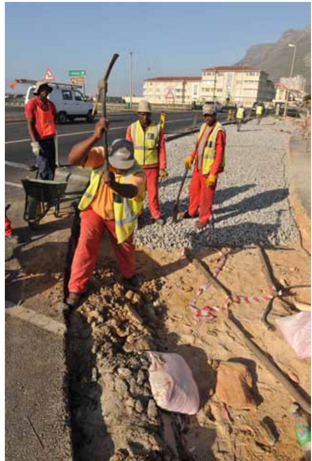
Roadworks in Muizenberg
